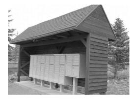
This component provides funding to stain and seal the wood mailbox covering. Wood slats are in excellent condition. Funding set based on observed condition.
