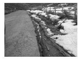
This component provides funding to repair erosion. The inspection found that runoff of the melting snow has carved 1' to 2' divots alongside the roads that are causing the edges of the road to crumble.
