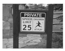
This component provides funding to replace the community's custom signage and  $6 \times 6$  posts as needed. There are 5 stop signs, 3 street signs, 3 "Children At Play" signs, and 1 "Steep Hill May Be Icy" sign. All were observed in fair condition and appear to have been replaced within the last few year.
