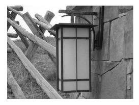
This component provides funding to replace the entrance lamps. They are made of metal and plastic were observed to be in fair condition.
