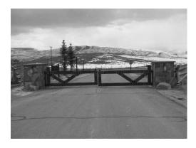
This component provides funding to maintain the entry gate. We recommend staining and sealing every 6 years. 14' x 4' and 4"" x 10"" wood beams with metal braces. Observed in good condition with no problems reported.
