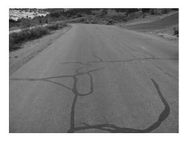
This component provides funding to crack fill. 312,000 SQ FT found in good condition overall. A few places that are crumbling. Mostly cracks that they fill each year.
